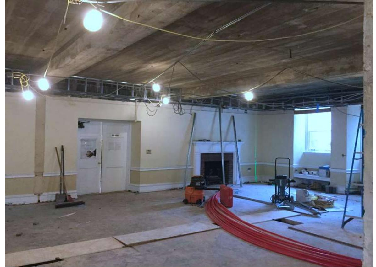
The bulkheads will hold ductwork and lighting bordering the higher center sections of the ceiling.
