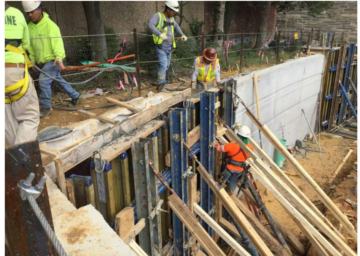
This completes the walls, so the wall forms can be taken apart and removed from the site, giving much needed breathing room for the other work.
