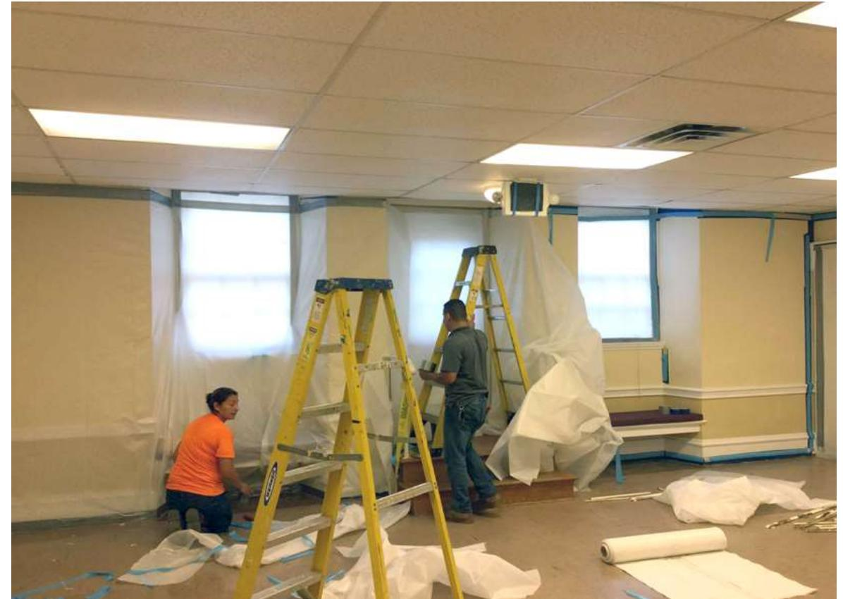
They wrap all the ducts and openings and install large filtered exhaust blowers to vacuum any stray particles out of the air and create a negative pressure environment.
