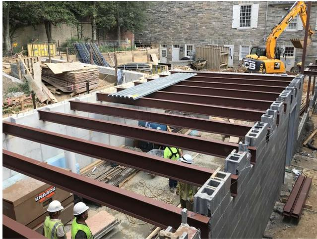
Now the beam pockets and bearing plates installed by the masons are put into service.
