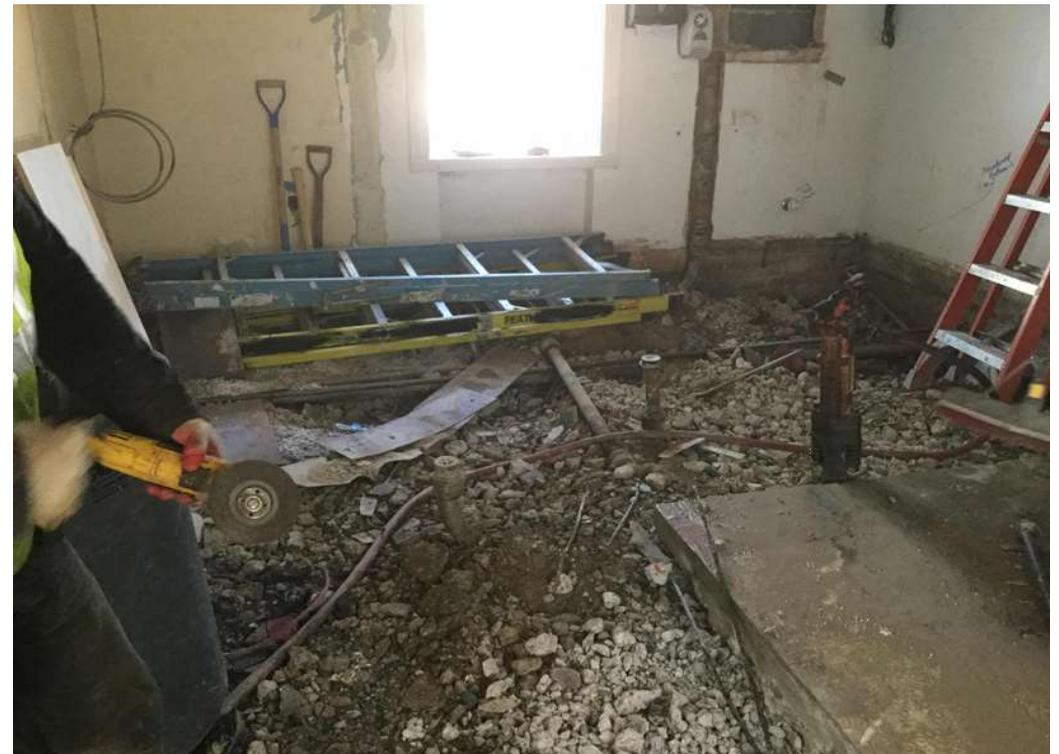
The plumbers come and cut and cap the plumbing and drains. An electrician reroutes electrical lines out of the way of the work.
