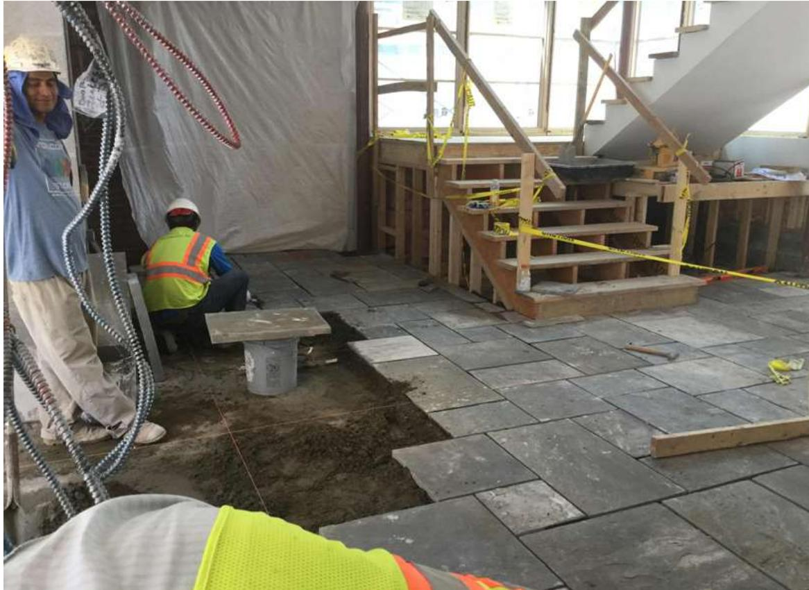
Douglas, Mario, and Tyrone (all of Monarc's own crew) clean up hallways, complete demolition of door sill number 14 (from the new corridor into the Carriage House ground floor offices), move scaffolding, install floor protection, and cut out a stone detail for the window sidelights.
