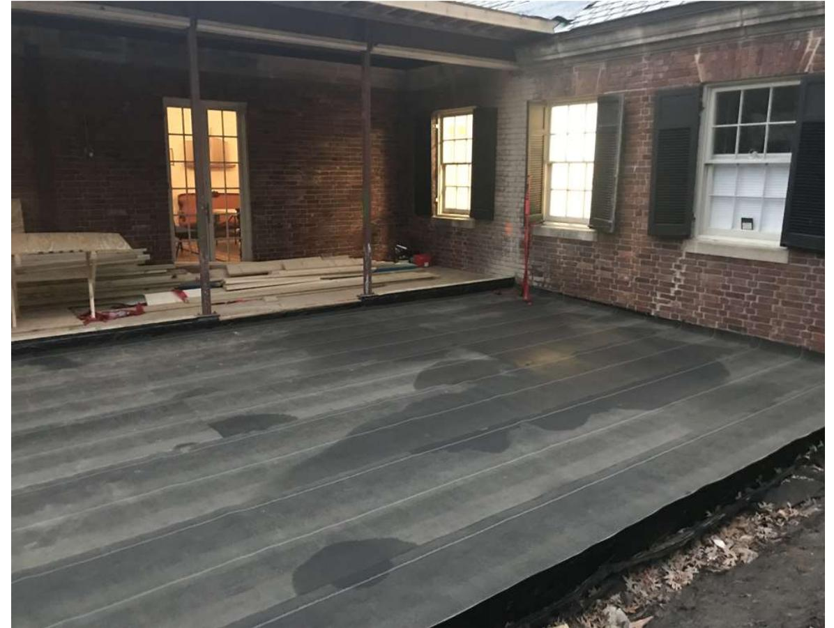
This protects the waterproofing layer below from damage as later material is added.
