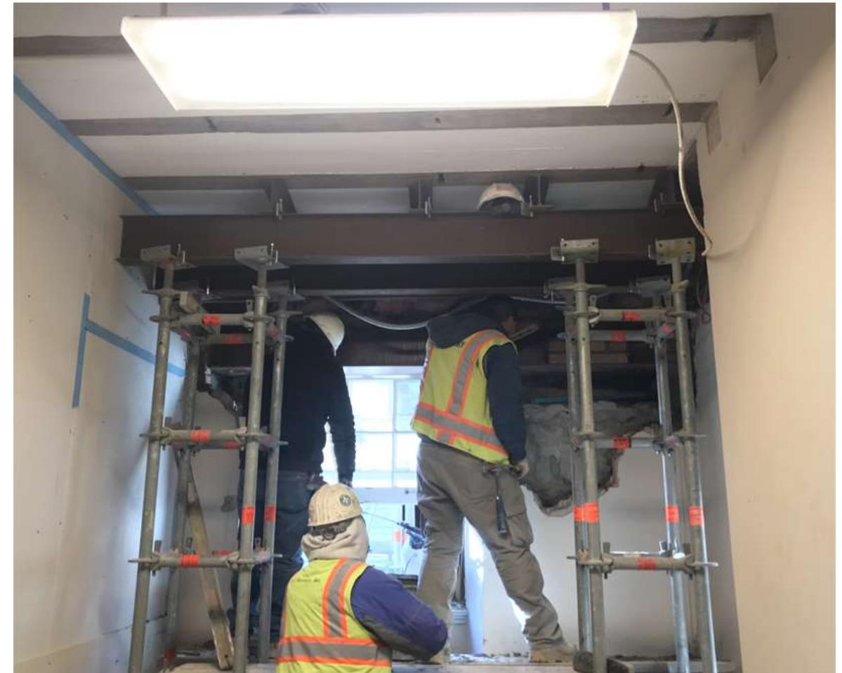
By the end of the day, the first lintel is in place and partly bricked in.
