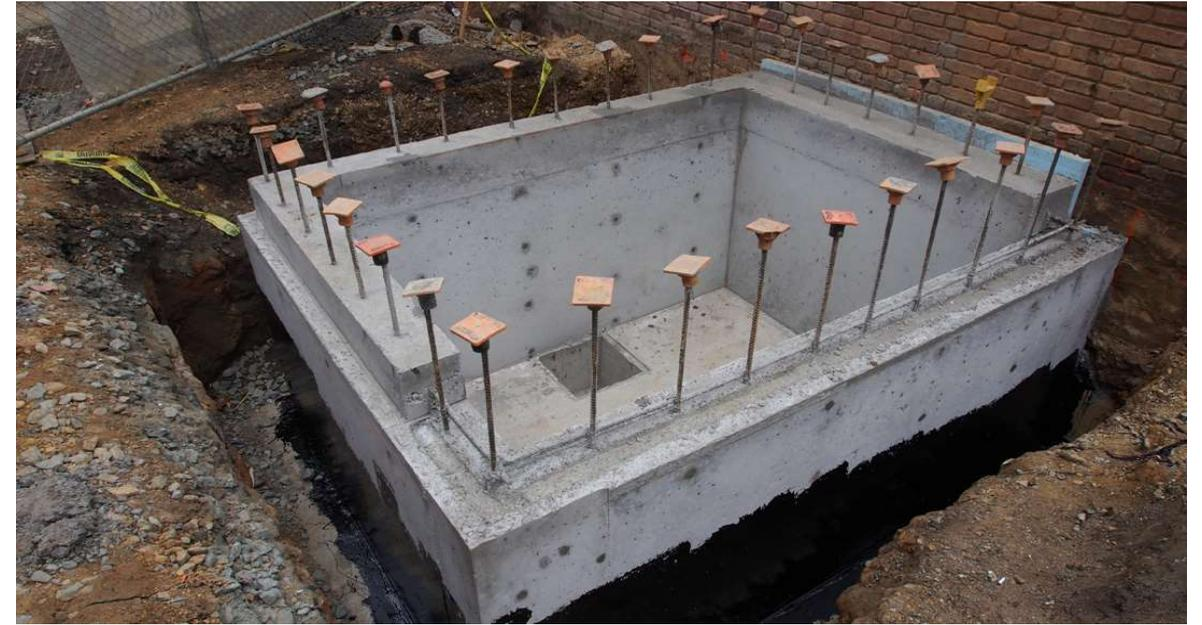
At the bottom of the pit, is a smaller, deeper pit. That's the sump, which is there to capture any water that makes its way into the pit (as it does in the basement of the Thai residency next door).
