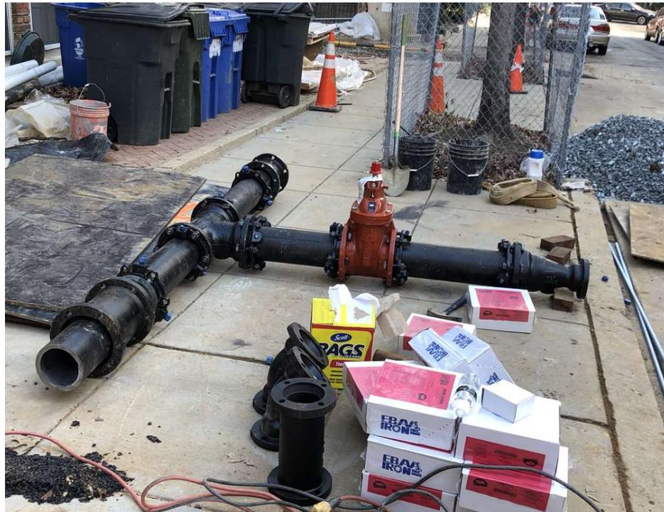
The red thing is the 6-inch valve that turns on the supply to our sprinkler system. The funnel on the right is a reducer that connects the 6-inch pipe to our 3-inch pipe. The crew has to cut a 10-foot section out of the DC water main and splice in the straight section of the T on the left.
