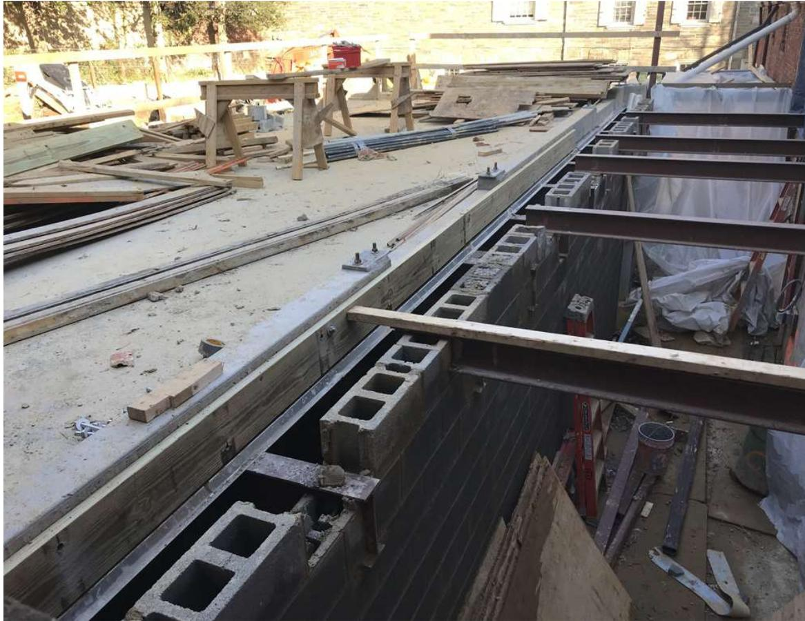
This sturdy piece of wood, now being bolted to the concrete upturn beam (which is also tastefully accessorized with bearing plates), marks the transition between the concrete Storage Room deck and the wooden Quaker House Living Room foyer floor.
