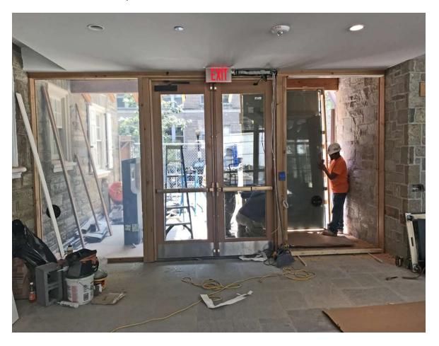
Work continues on repairing the holes left by the removal of the Carriage House stairs and office walls.
