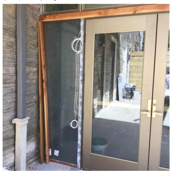
Installation of the sidelights is slowed by the need to rechannel the frames to accommodate the inch-thick glass.
