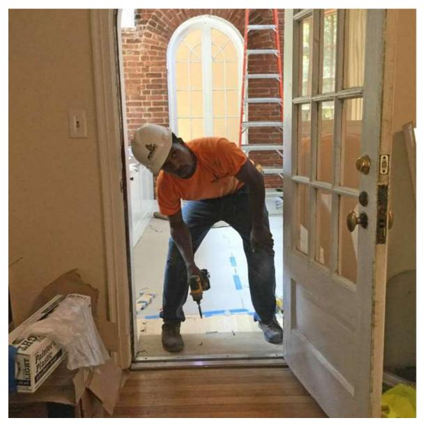
Tyrone, Mario, and Douglas work on threshold and floor transitions and interior paneling, and then start to frame a new floor to cover the departing stairwell in the Carriage House west office.
