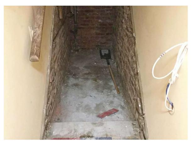
They discover that the space below, which is to become a large utility closet, has a dirt floor, so additional work will be required to extend the slab into this area.
