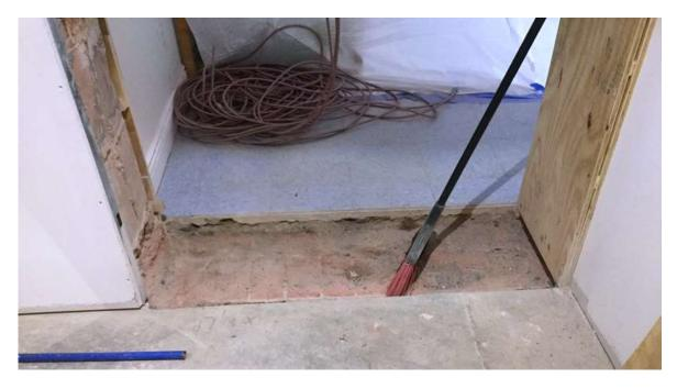
Four electricians turn off all the power in Quaker House and Carriage House and connect them to the new main panel in the Storage Room. They also install conduit for floor boxes in the Lobby.
