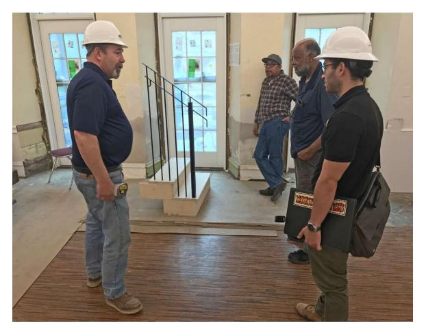
This is a mockup of the planned Lobby stairs, created by the ironworkers and carpenters, so the architects can approve the details before construction.
