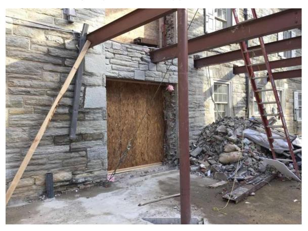
The guy wire helps to hold the Lobby steel where it should be until the ironworkers come to weld it into rigidity.
