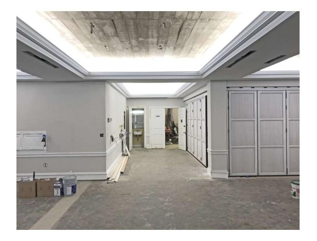
Ceiling installers arrive up to install 900 square feet of fabric-covered acoustic ceiling in five Assembly Room bays. They are surprised to discover that they are expected to attach the ceiling to a 90-year-old concrete slab. They depart, promising to return with the proper fasteners.
