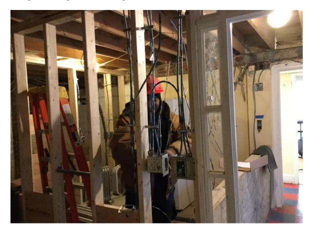
The ceiling crew finishes laying up the plywood strips and adds metal framing, into which the fabric ceiling will be tucked.
