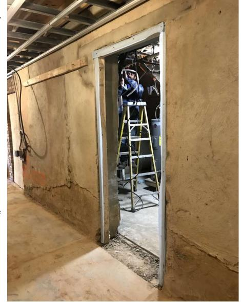
Carpenters add some framing to support the new Carriage House roof.
