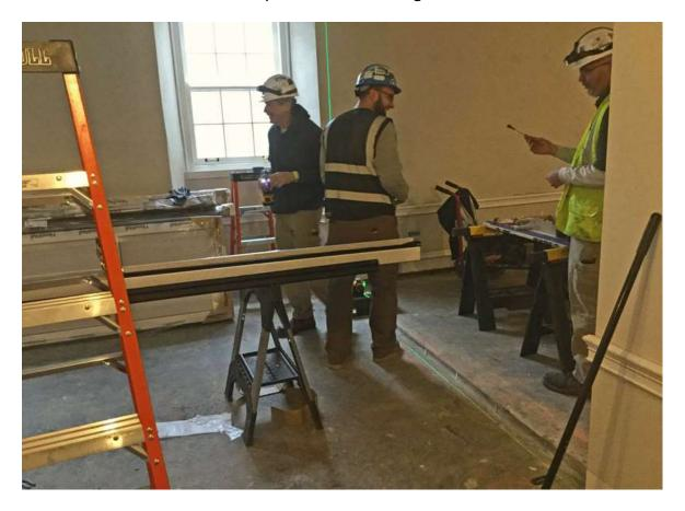
Also in the Assembly Room, electricians start to install nearly 300 feet of LED lighting above the crown molding.
