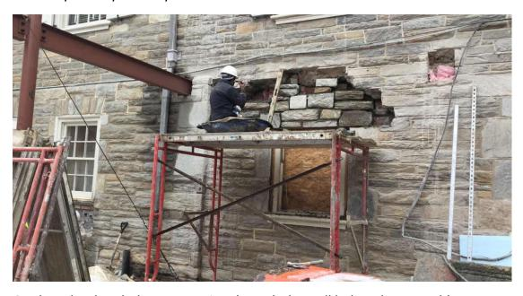
On the other hand, they are sawing through the wall below the Assembly Room doors and windows and chipping away at the stone.
