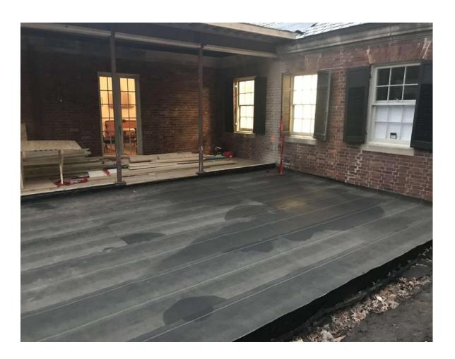
This protects the waterproofing layer below from damage as later material is added.
