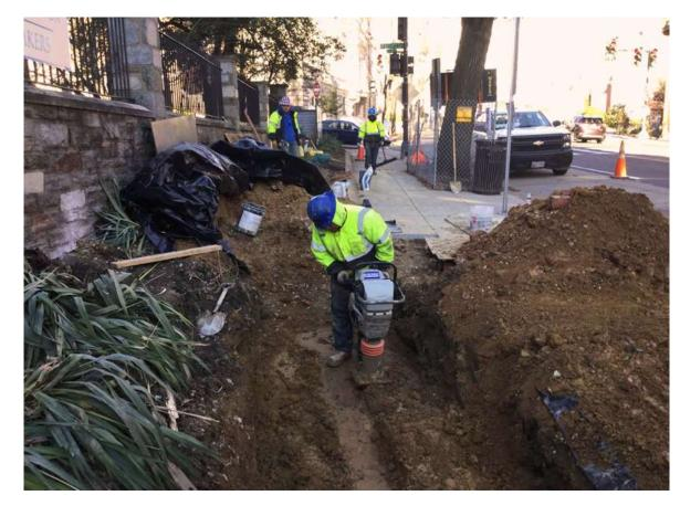
The next step is to move inside the garden, dig a large hole, and connect it under the wall to the manhole.
