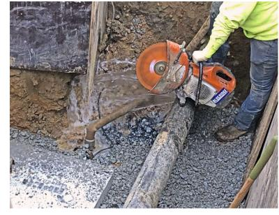
With a pump running, they splice in the new section.
