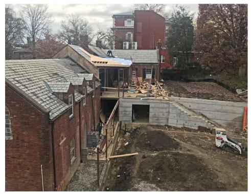
As darkness closes in, with rain in the forecast, a lonely roofer installs temporary roofing on the new wood.
