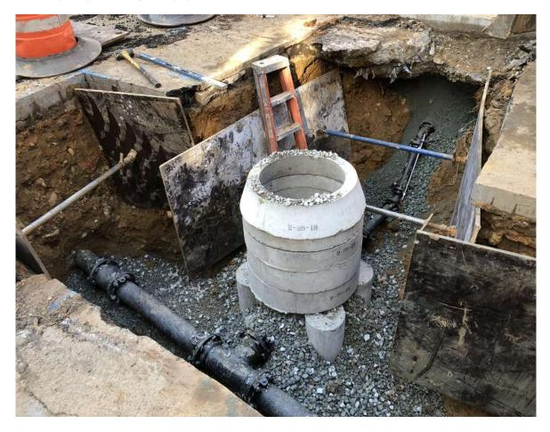
The valve rests on a concrete base, which they top with four round spacers and a round access hole, so future generations of plumbers can turn our supply off when needed.
