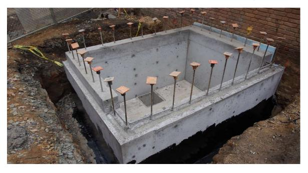
At the bottom of the pit, is a smaller, deeper pit. That's the sump, which is there to capture any water that makes its way into the pit (as it does in the basement of the Thai residency next door).
