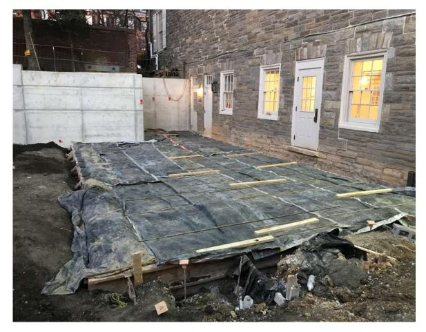
Concrete produces heat as it sets, so it will keep itself warm enough. They had a blanket on the area the night before, as well, to keep the ground from getting too cold overnight. The concrete crew also prepares for one more pour at the new west stairs — a slab to connect the bottom of the new stairs with the top of the old.
