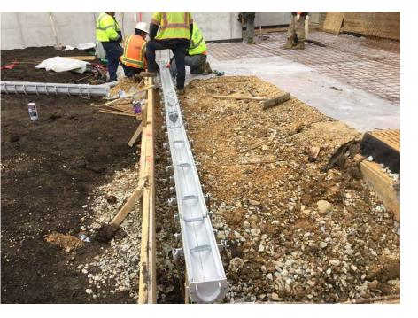
They also install the last drainage connection to tie new downspouts into the new drainage system.
