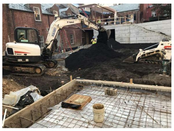
while steel mesh is installed around the drains to reinforce the new patio.
