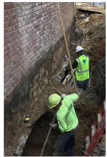
The underpinning begins with the digging of several holes under the Carriage House east wall.
