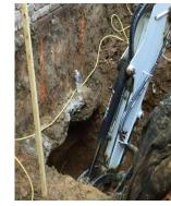
No pins are involved. The concrete crew digs a hole under a few feet of the existing foundation and pours a newer and deeper foundation, then moves a few feet and repeats the process until a whole section of the building is done.
