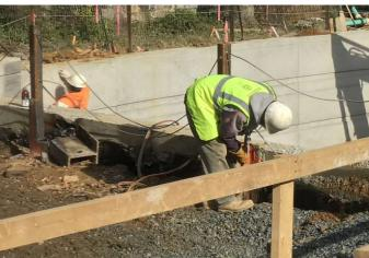
Carpenters continue to install ledger board and pad the tops of the steel beams to support floor joists.
