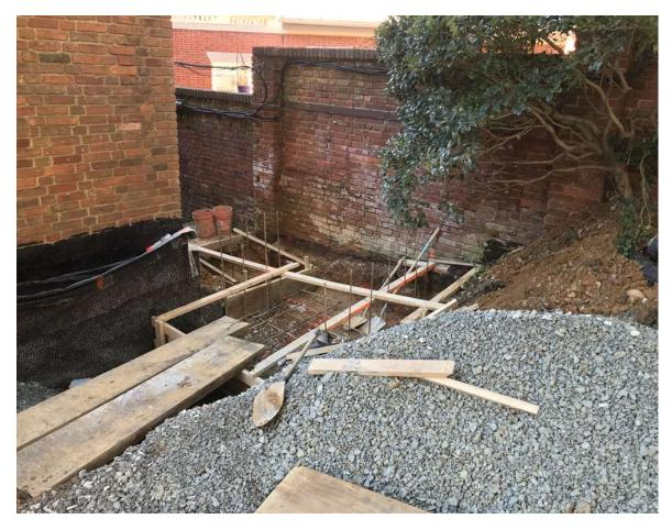
The black waterproofing on the wall shows where the new ground level will be. The orange buckets show where the bottom of the stairs will begin.
