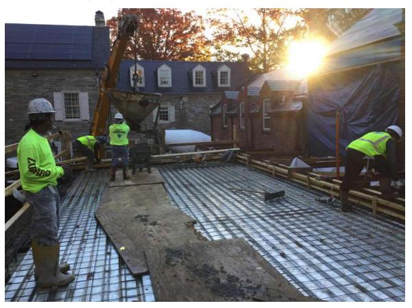
The concrete crew pours the roof of the Storage Room, which now also possess four walls and a floor. Almost a room.
