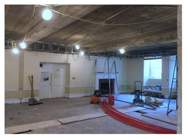
The bulkheads will hold ductwork and lighting bordering the higher center sections of the ceiling.
