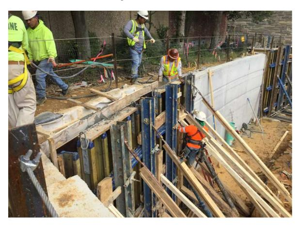
This completes the walls, so the wall forms can be taken apart and removed from the site, giving much needed breathing room for the other work.
