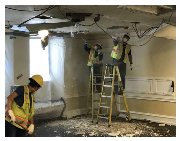
They start to remove that, but then notice that it was glued in place and declare that the old glue has to be tested for asbestos before they can continue.
