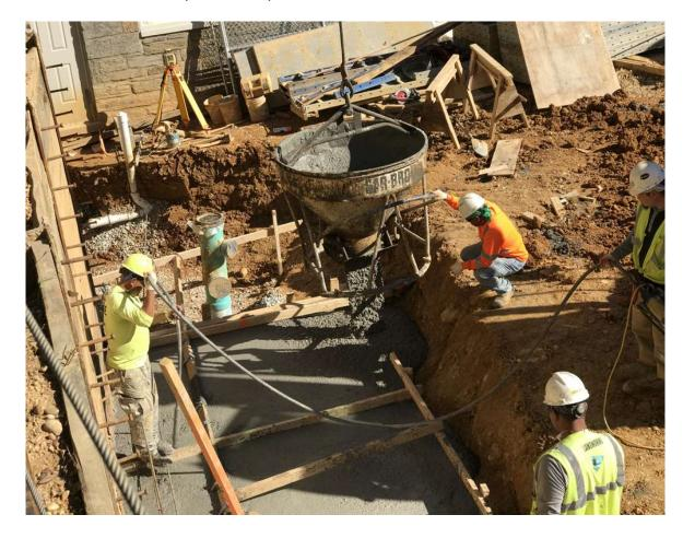
The wall is not designed to have a foundation, but the concrete crew feels they want one to stabilize the complex wall forms in the next step.
