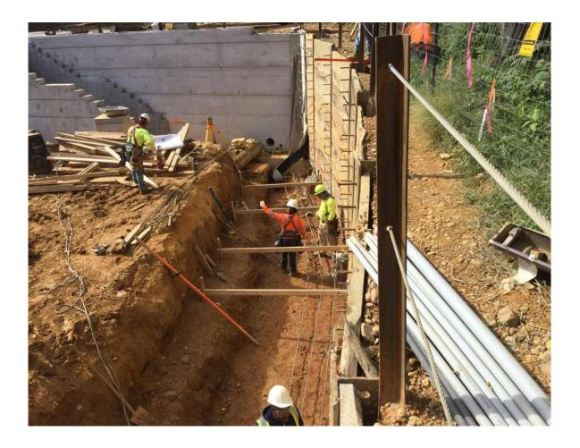
A dozen concrete and shoring workers ready the foundations of the curved wall for tomorrow's pour, laying steel, setting forms, extending shoring, installing more Nelson studs.
