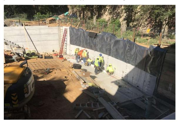
Nine concrete workers start to lay out the steel and wall panels for that wall.
