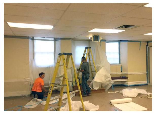
They wrap all the ducts and openings and install large filtered exhaust blowers to vacuum any stray particles out of the air and create a negative pressure environment.
