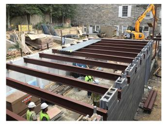
Now the beam pockets and bearing plates installed by the masons are put into service.
