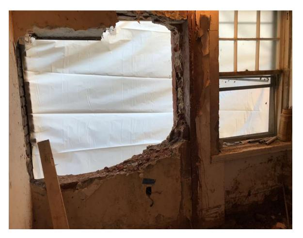
The picture window on the left will be the hallway from the corridor to the Quaker House man stairs. The window on the right will be the doorway from the corridor to the new ADA bathroom.
