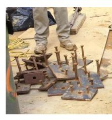
The masons, practically every day, are also installing bearing plates to hold the steel beams that will carry the floors of the upper level.
