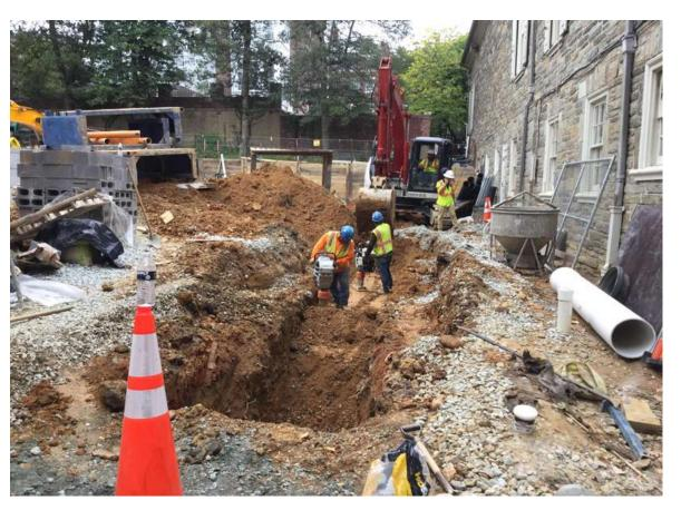
Although you will never see that pipe, it is very important, as it goes under the Lobby to the street, and it's the only way for water falling on the back garden or coming down from the Costa Rica Embassy drain to get out of our enclosed yard. It's either through the Lobby or under it. Nine concrete workers are also here, and they are busy preparing to pour the other side of the stairway. The masons have also been at work here.
