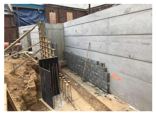
The masonry wall on the right will support the right side of the stairs. The forms on the left will form the concrete for the left side (coming down). You can faintly see the junction boxes for the lights, marching down the wall. The black form panels are the place where the stair reaches a landing and turn right, out onto the lawn.
