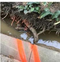
One way to handle them would be to dissect them out of the soil with an air knife and then install the new pipe underneath them and put the dirt back.
