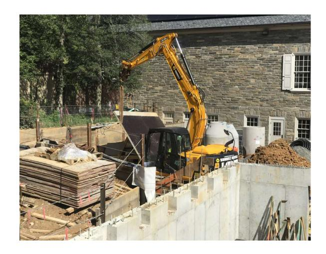
It drops a trench box into the hole to protect against wall collapse.
