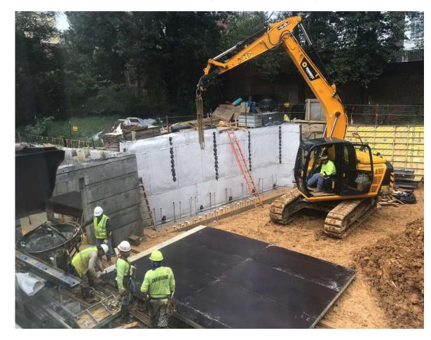
The wall will be poured against that, backed up by the drainage board.
