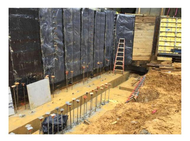
The drainage board (magnified at right) is plastic and full of holes that capture water that comes through the soil and channel it down the wall.
