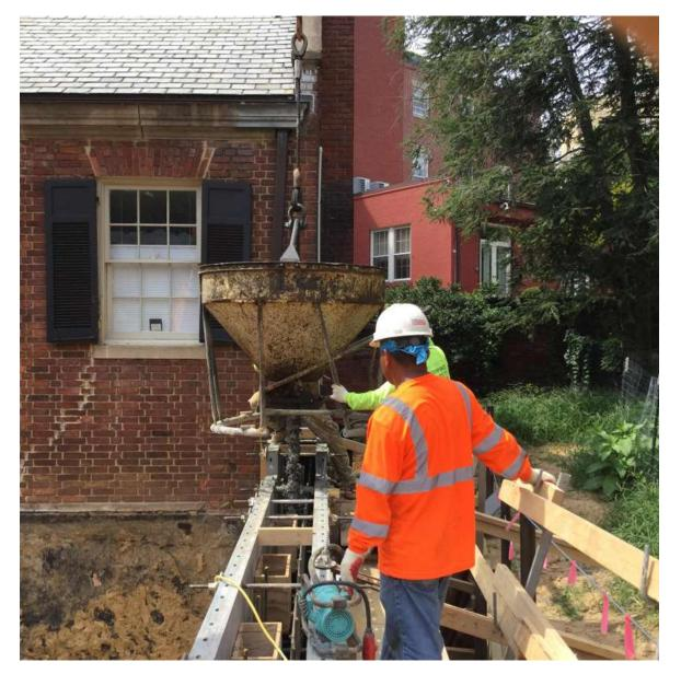
Notice the little boxes at the top, inside the form? Those are beam pockets that will hold the other end of the support beams.
