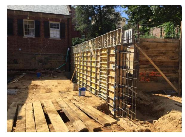
The concrete will be poured over the reinforcing steel between the metal panels.
