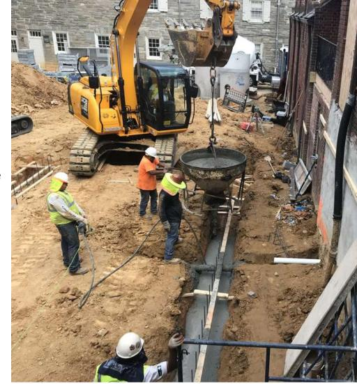
The pipe running across the footing is a new drain pipe from the soon-to-berenovated Quaker House Boiler Room.
