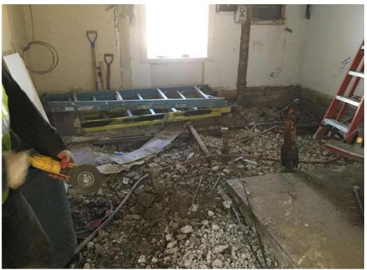
The plumbers come and cut and cap the plumbing and drains. An electrician reroutes electrical lines out of the way of the work.
