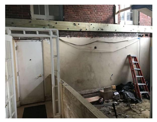
Here, you can see the new sill plate bolted across the wall, which will support the new floor. You can also see the beginnings of the pedestrian walkway on the left for use by our tenants during the work.
