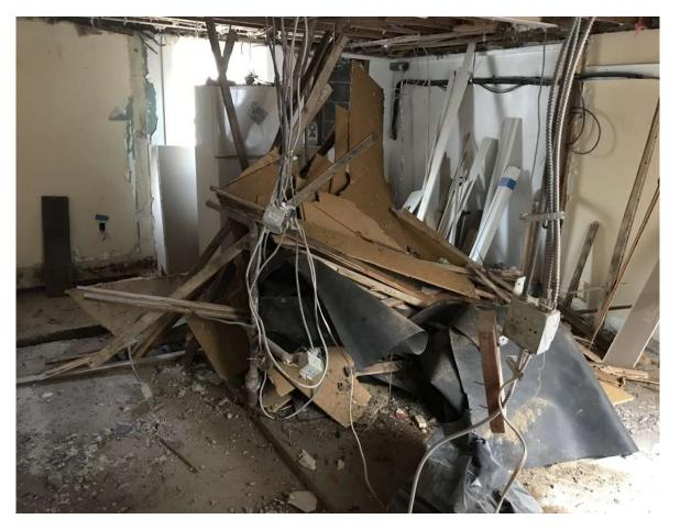
Up above, the decking is torn off, along with underlying roof membrane, so a protective tarp is added to keep the rain out.
