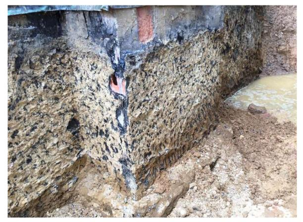
We need to do that, because the ground at this point will be built up to the higher level of the new Quaker House Terrace and that could cause new water issues. There will be a new foundation drain here to help keep Quaker House dry.
