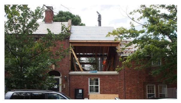
They also install roof jacks (just to the right of the roof in the above picture) to support a platform so they can temporarily relocate the heat pump compressor (now on the deck) to provide continued service to Carriage House during the work.
