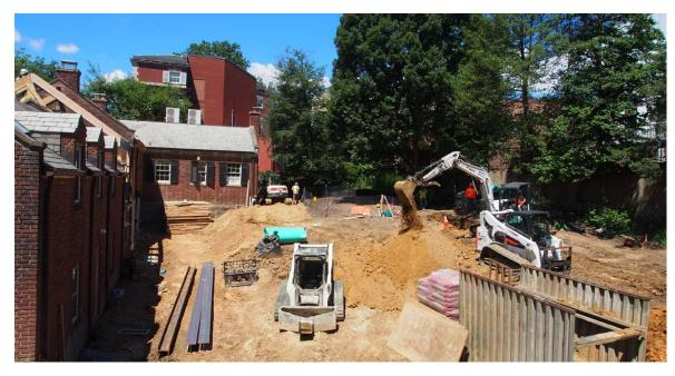
In the upper left, carpenters continue to frame the new roof over the Carriage House deck. On the right, excavators dig a trench for an 8-inch drain line that will serve drains on the upper terrace.
