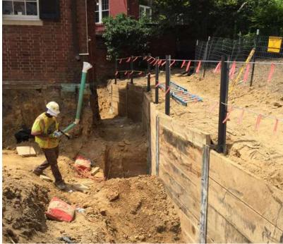
Excavation and installation of new drains continues . . . The lagging (wooden cross-pieces) are inserted between the pilings (vertical steel beams) to hold back the dirt as they dig down. A cable safety railing is installed as the new levels emerge.
